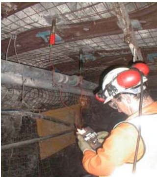
Testing rock bolts with the RF System in a coal mine
